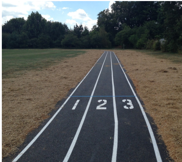
The new track at Lincoln Elementary School.
